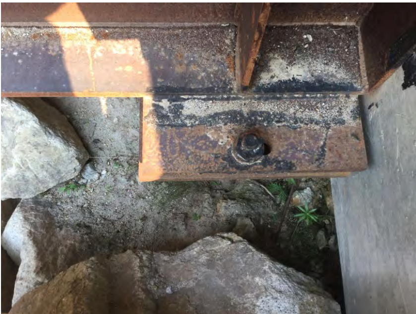
Bolts at extent of slots at right abutment
