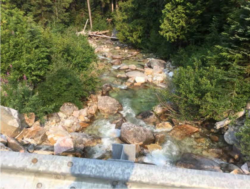
Looking downstream from deck
