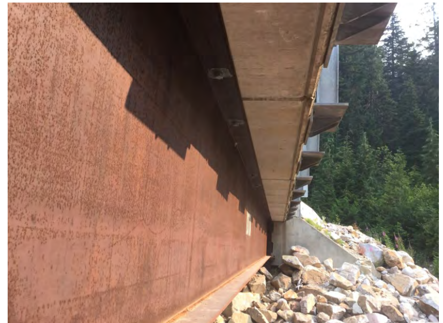
Deck bolts - typical
