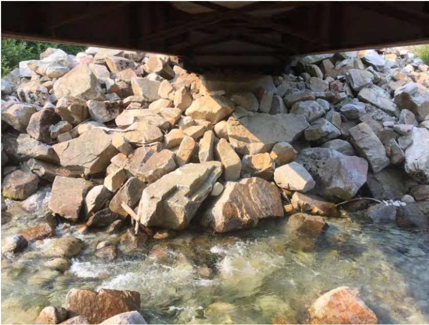
Left Bank Abutment when facing downstream
