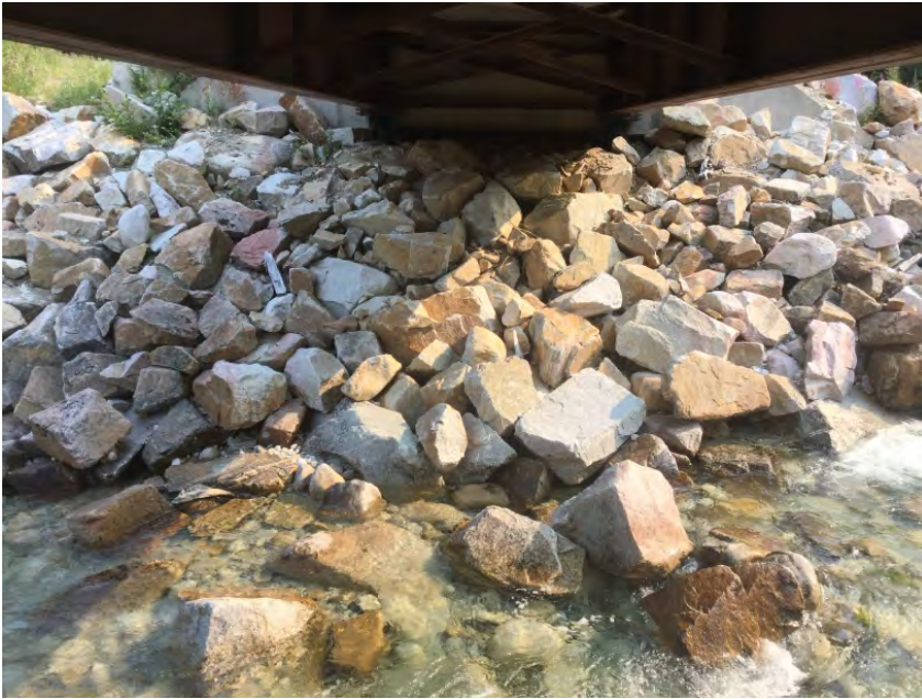
Right Bank Abutment when facing downstream
