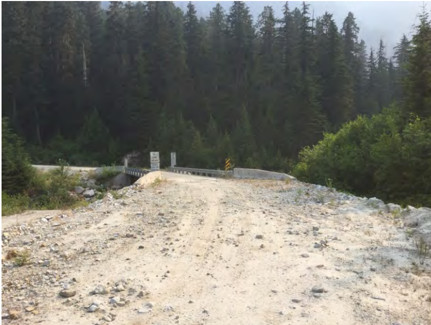
Approach from Left Bank when facing downstream
