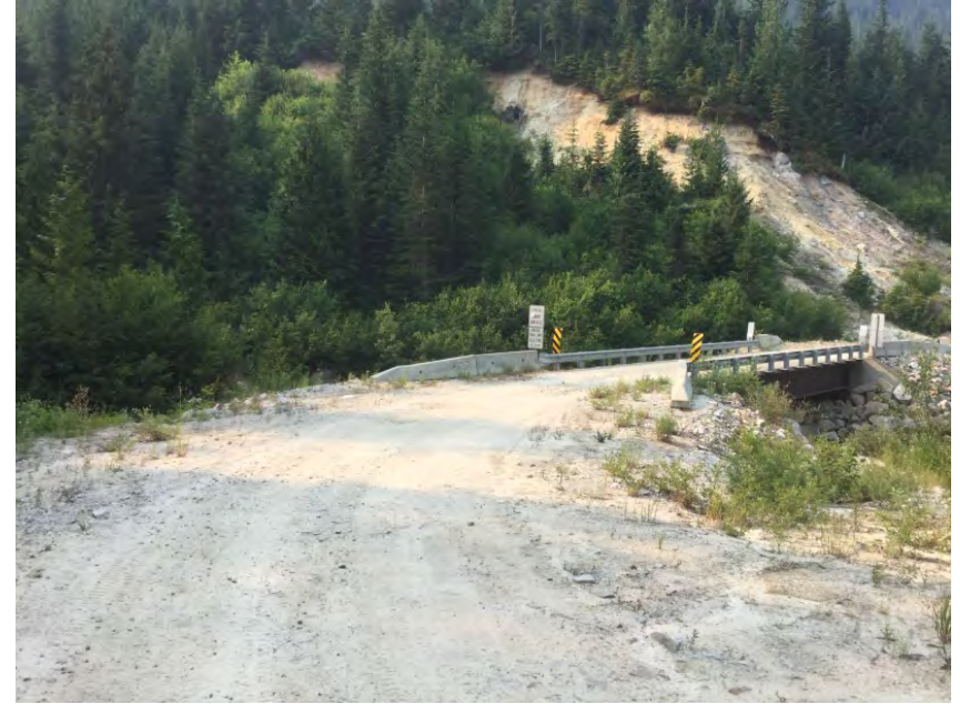
Approach from Right Bank when facing downstream
